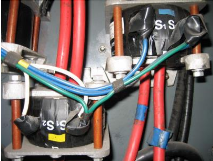
Figure 1 Incorrect CT Orientation
